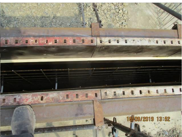
Photo: Shuttering at the retaining wall.
