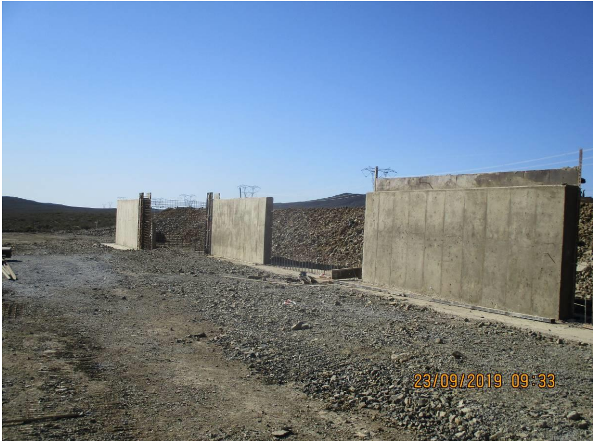
Photo: Retaining wall in progress.
