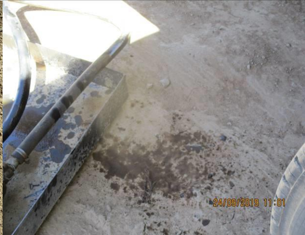
Photo: Diesel spill at the refuelling area.
