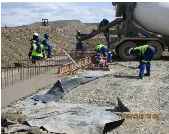
Photo: Concrete work at the retaining wall.
