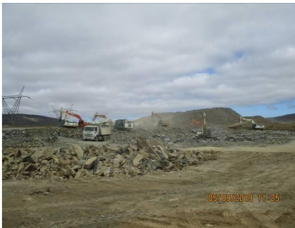
Photo: Breaking of rock at section D.
