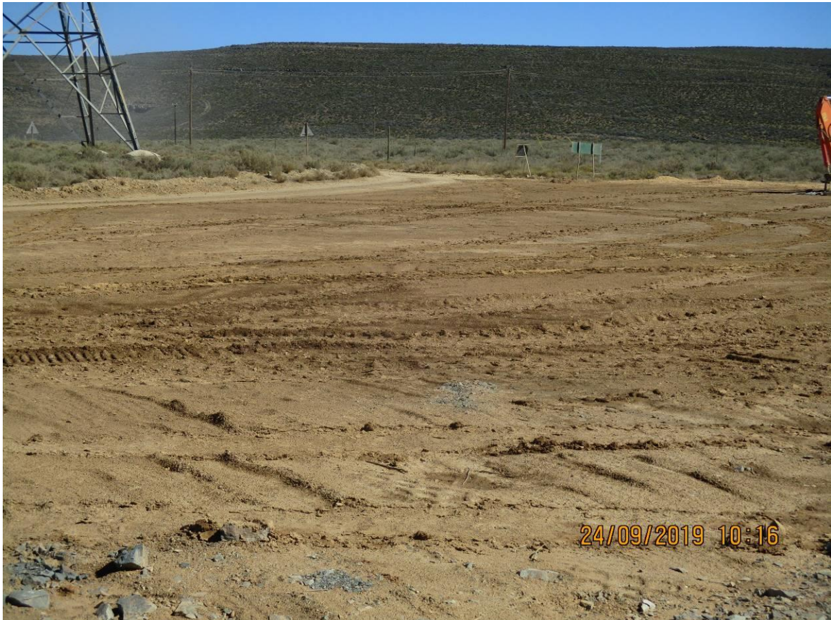
Photo: Dust suppression implemented at the heavy machinery parking area.
