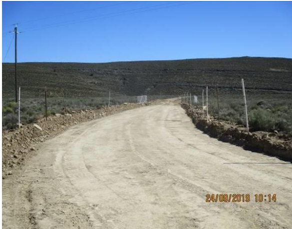
Photo: Road bed on permanent road.
