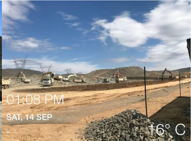
Photo: Road bed preparation at section D1.
